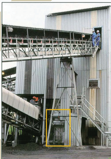
The Spirotech sampling plant compared to the old sampling tower
